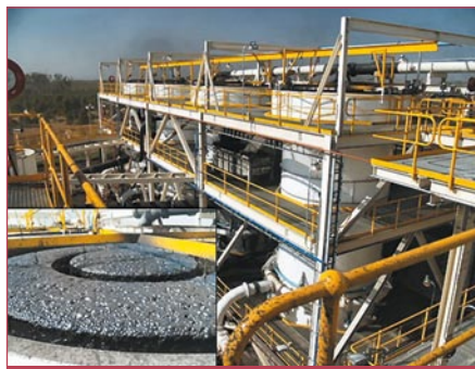
Figure 19. 4.9 m (16 ft) diameter by 12.8 m (42 ft) tall column flotation cells with froth product shown (inset).
