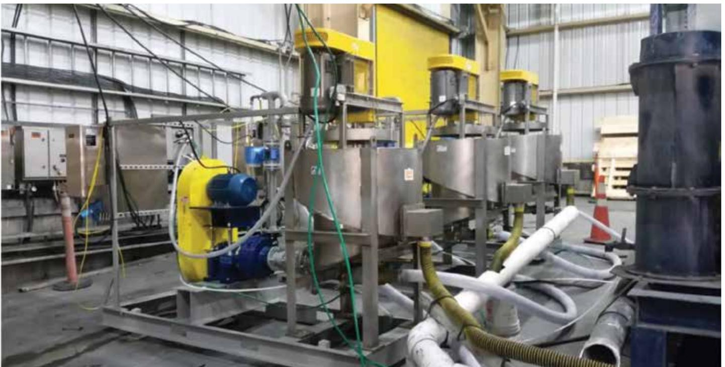
**Figure 3: A train of three 0.6-metre StackCells used in this evaluation.**
