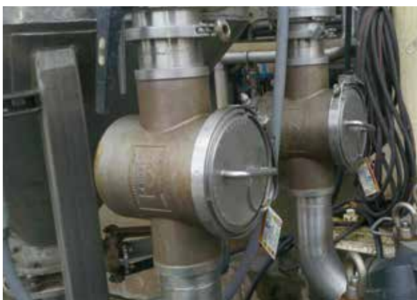
Magnetic traps are ideal for removing tramp iron contaminants in liquid line applications.
